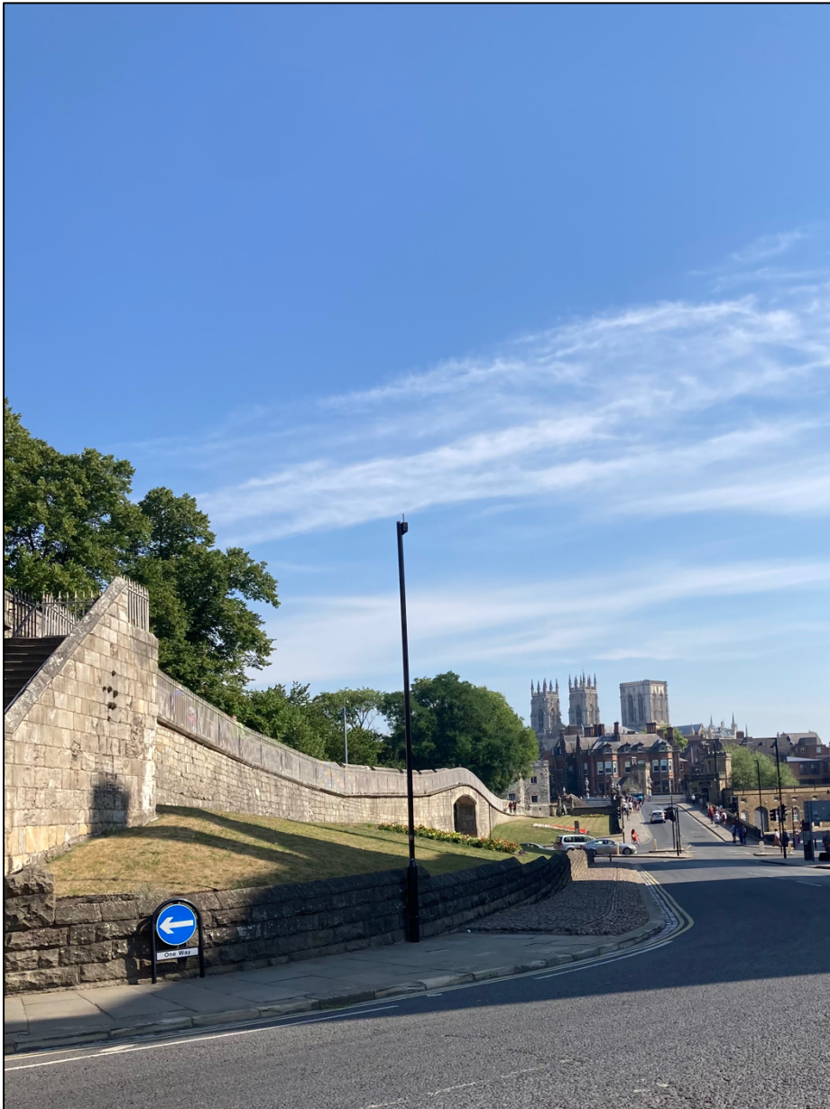
Figure 1 - The city walls of York before entering the historic core (Source: Researcher's own photo)
