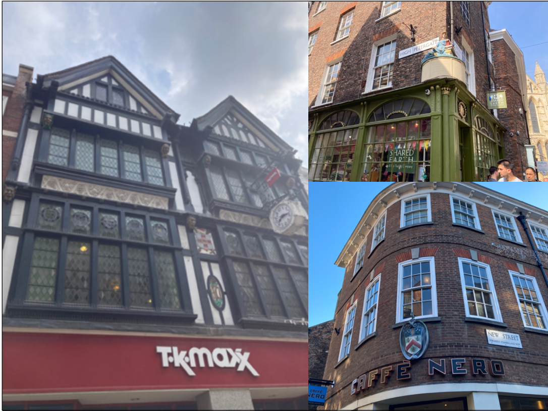
Figure 14 – Distinctive shop architecture, with symbolic markers - lining the streetscapes of the historic core. (Source: Researcher's own photos).
