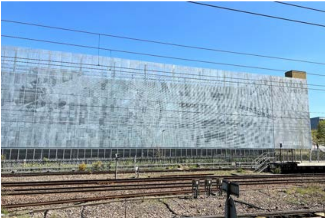
Figure 36: Station Gateways new multi-storey carpark, 'advertising' the town's contribution to aerospace engineering (Researchers own, 2023).
