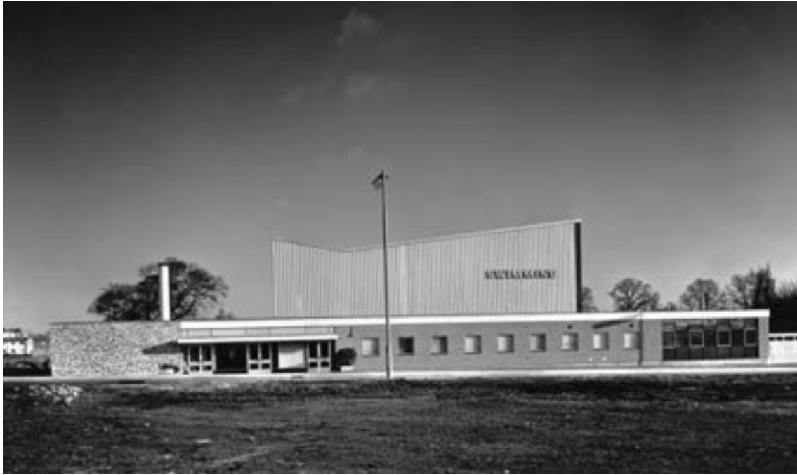
Figure 39: Stevenage Swimming Pool exterior in 1963 (Pantlin, 1963).
