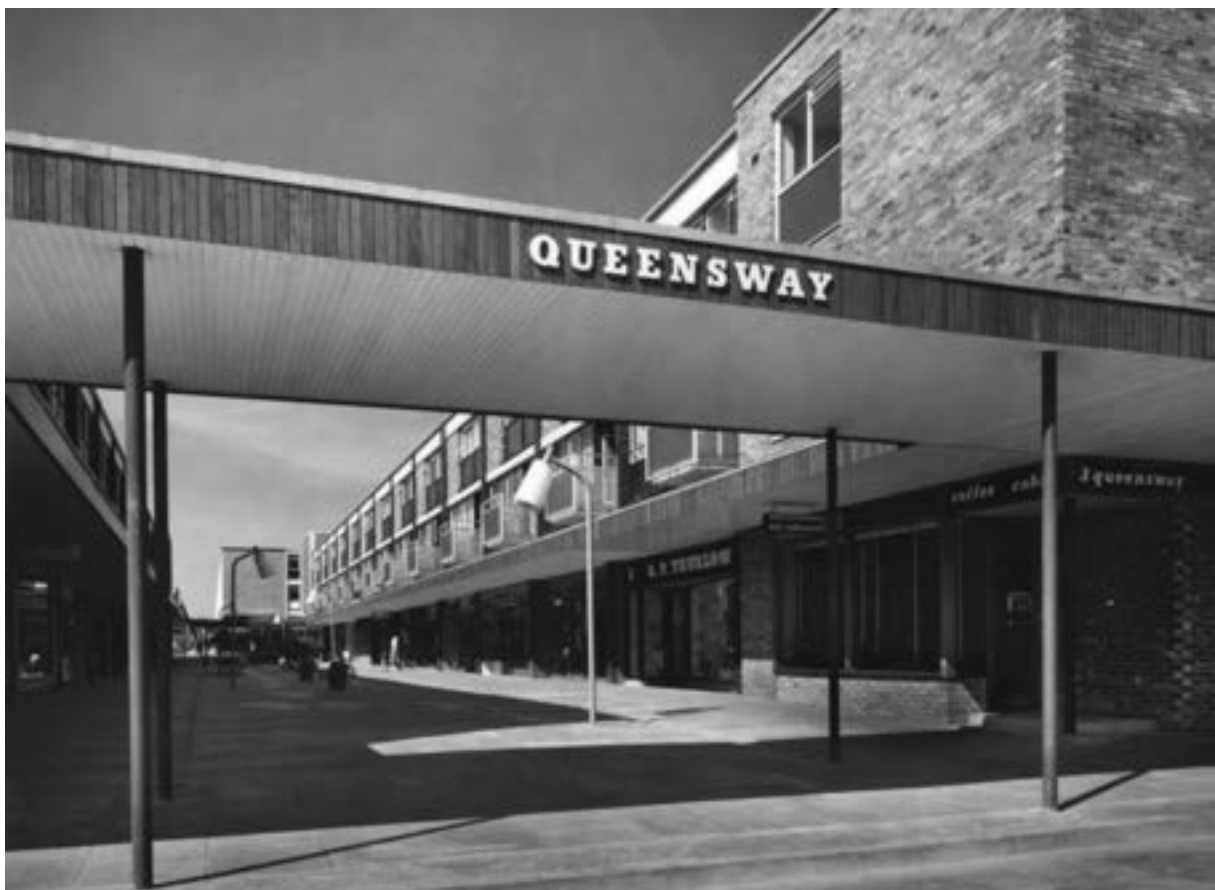
Figure 15: View looking north on Queensway – Stevenage’s primary north-south pedestrianised avenue – in 1959. The timber-finished canopies were a key design element of the Centre; enabling architectural uniformity, visually separating the street from the building above and providing shelter (Maltby, 1959).
